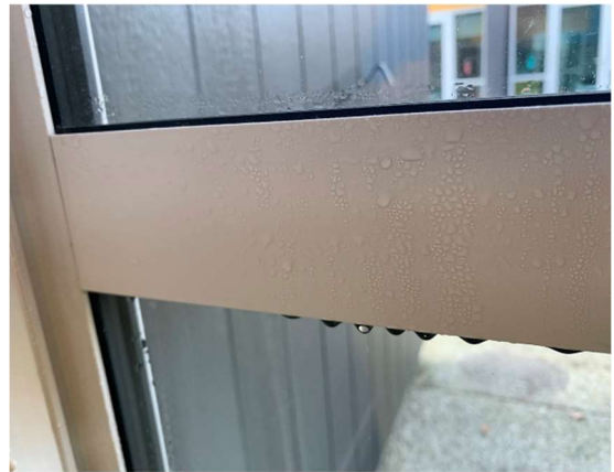
Figure 1: Waikato - Double Glazed Non-Thermally Broken Joinery
