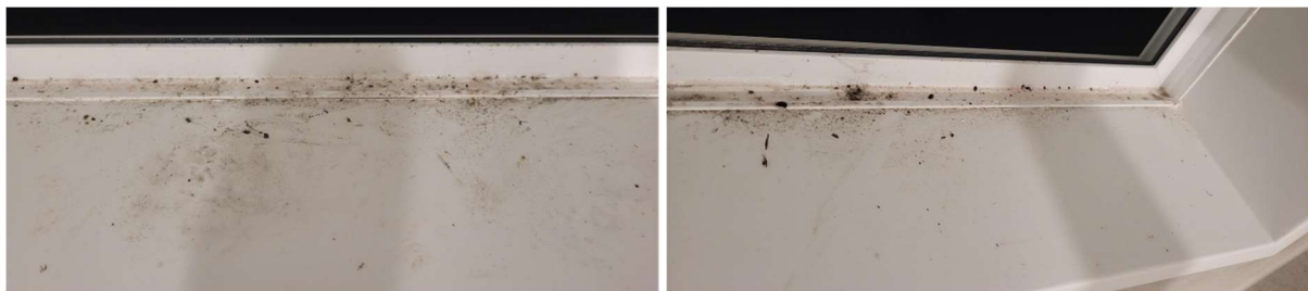
Figure 2: Auckland Residence - Homeowner actively attempting to use natural (window) ventilation while maintaining indoor air temperatures, still resulting in mould
